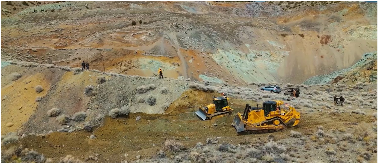
Picture 2 – PUF and backfill permanent closure of two hazards at the Olinghouse Hard Closure Project in Washoe County, NV
