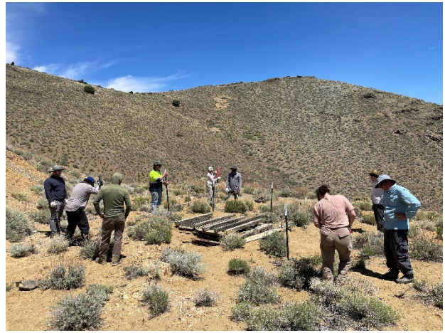
Picture 3 – Summer interns securing a deep mine shaft in Washoe County, NV,
